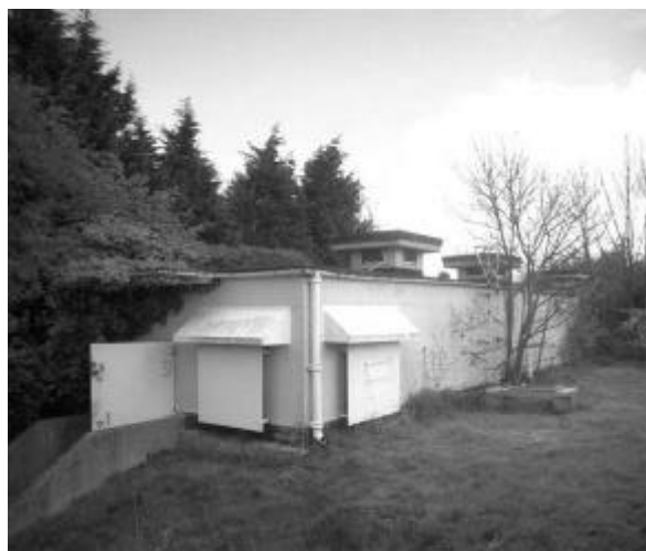
Surface entrance to Watford Group HQ
